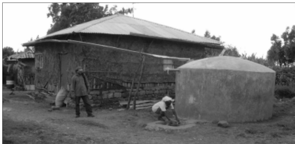
Figure 2: Typical wattle-and-daub building in Ethiopia with large ferrocement tank
