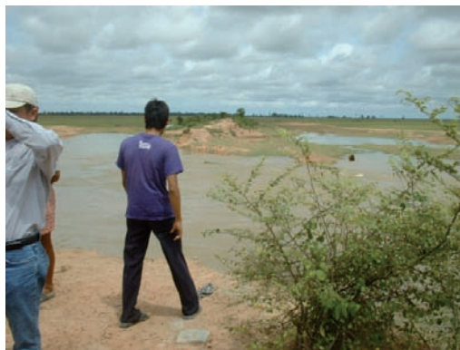
Breached embankment that no longer stores water for use later in the dry season. With each rain season, the breach gets wider.
