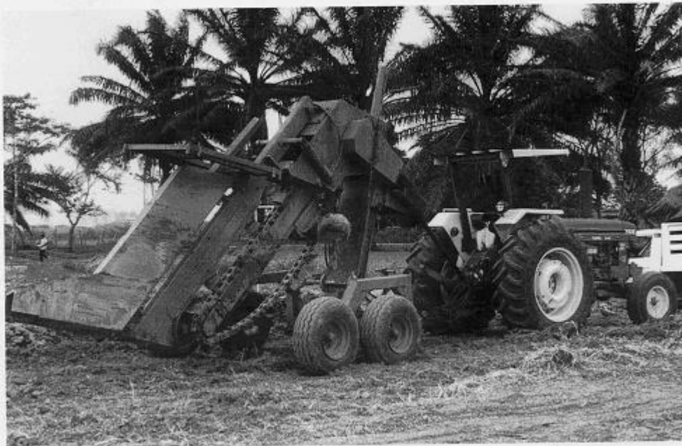
Photo 2 Tractor-drawn drainage machine with chain box
